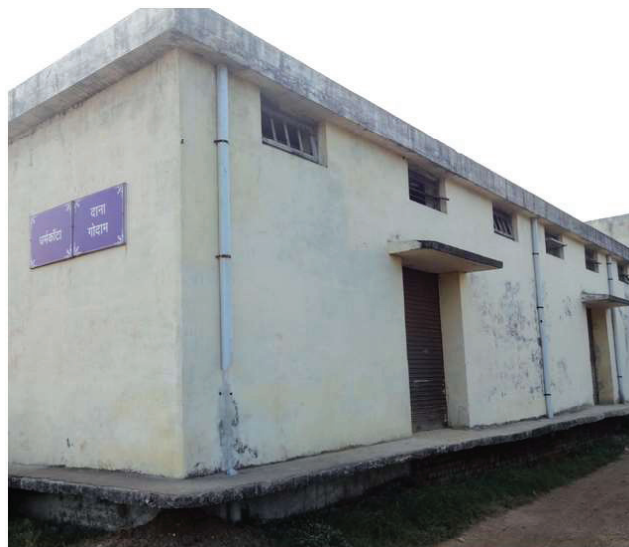
Fig. 4.15: Feed godown on raised platform
