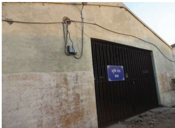
Fig. 2.29: Entry of an implements shed
