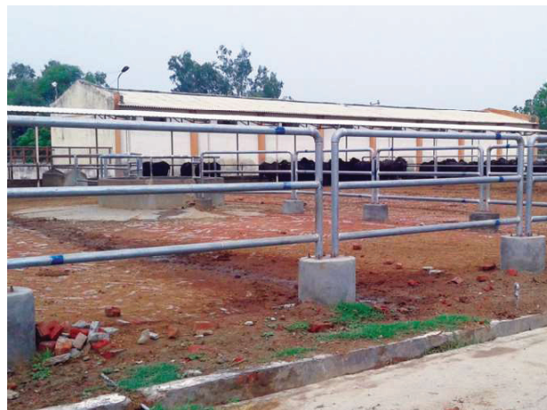
Fig. 2.5: A view of loose housing for livestock
