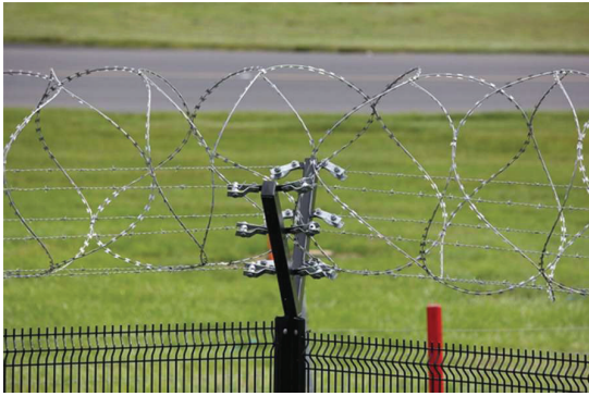
Fig. 4.6: Barbed wire and electric fence
